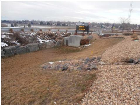
This stormwater detention pond and inlet is located at the Apex Field House at 58<sup>th</sup> and Oak Street. The detention pond detains stormwater to settle out contaminants before discharging, letting a portion of it infiltrate. Detention ponds like this one are found throughout the City and help aid in settling out sediment in stormwater prior to it entering our waterways.
