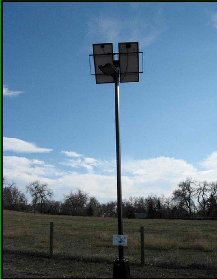
Solar LED Lighting
